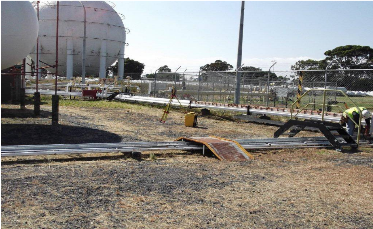
Location of Elgas plant where the gold pipe stands were installed
